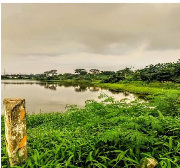
Plate 5: Restored Awba dam (University Ibadan)
