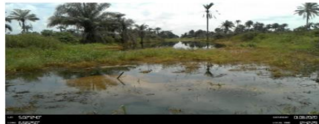
Overview: Part of spill impact on 14" Okordia - Rumuekpe Pipeline at Edeoha. Picture was taken during Joint Investigation of 1 st Aug 2020.
