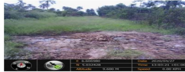
Overview: Part of spill impact on 14" Okordia Rumuekpe Pipeline at Edeoha. Picture was taken during Joint Investigation of 27 th April 2020.
